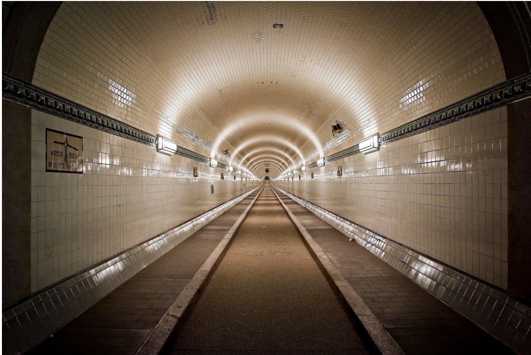
Figure 14. One of the two tubes of St. Pauli Elbe Tunnel. [Photographed by Markus Daarms (Pixabay)]
