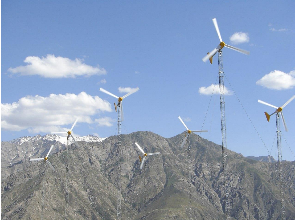
FIGURE 1 Afghanistan's first wind farm in 2008: 10 turbines in Panjshir Valley. The windfarm was installed by Empower Consultants in NZ and delivers 75 kW of electricity for government facilities in the Panjshir Valley (Scoop Business, 2008). Photograph by Daniel Wilkinson (U.S. State Department), U.S. Embassy Kabul Afghanistan, Public Domain ( https://commons.wikimedia.org/w/index.php?curid=22226462 )
