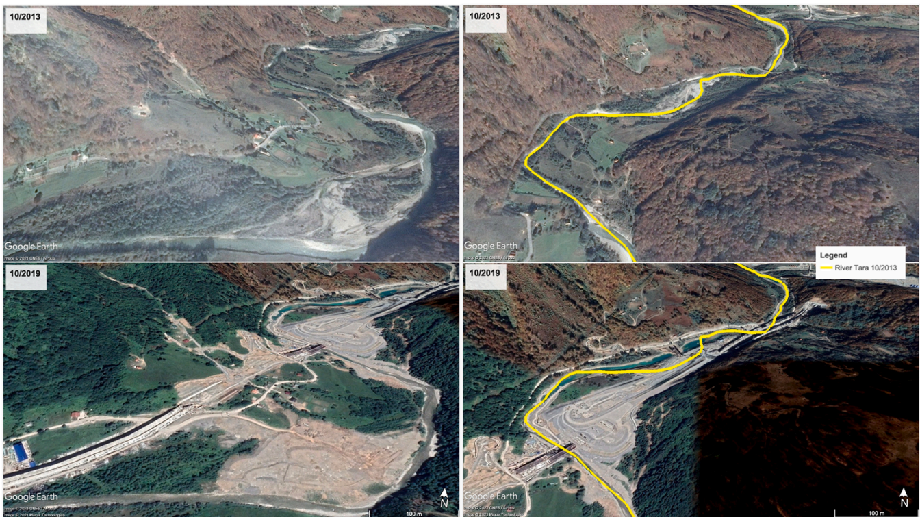
Fig. 3. River Tara before and after the highway construction started near Mateševo. Bottom left: materials disposed close to the river. Bottom right: modifications of the river course.
