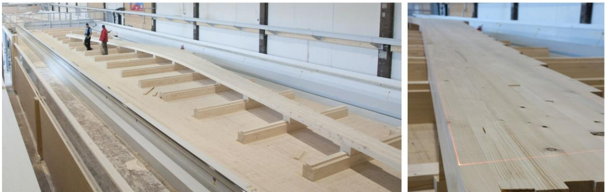
Figure 35: Industrial wood truss production (with courtesy of LAP GmbH Laser Applikationen)
