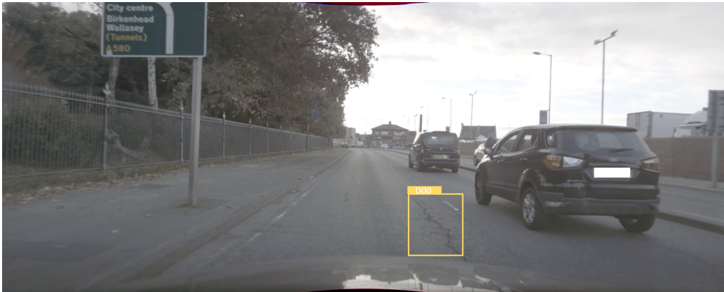
Figure A.4: Longitudinal crack (D00) in an example image of the ADS (UK)
