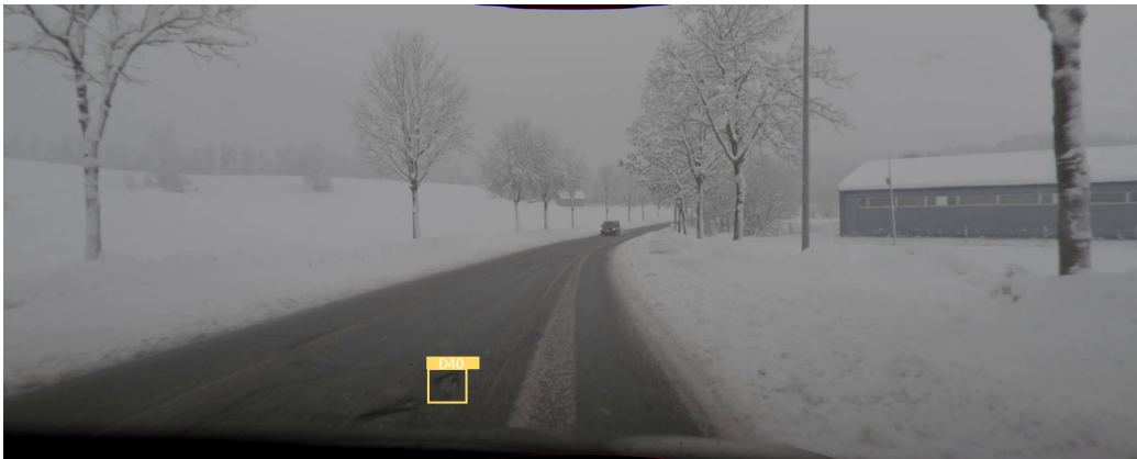
Figure A.8: Pothole (D40) in an example image of the ADS (Germany)
