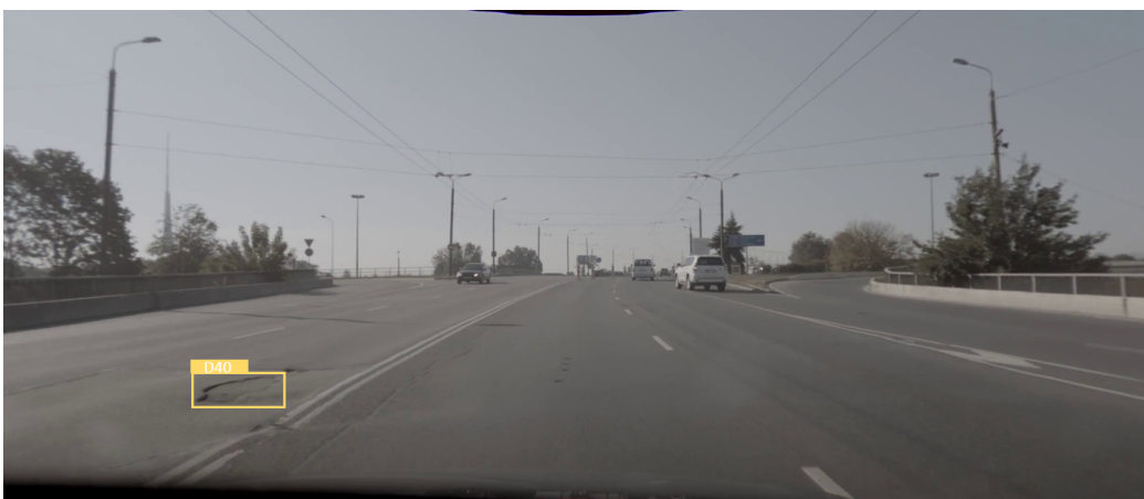
Figure A.6: Pothole (D40) in an example image of the ADS (Latvia)
