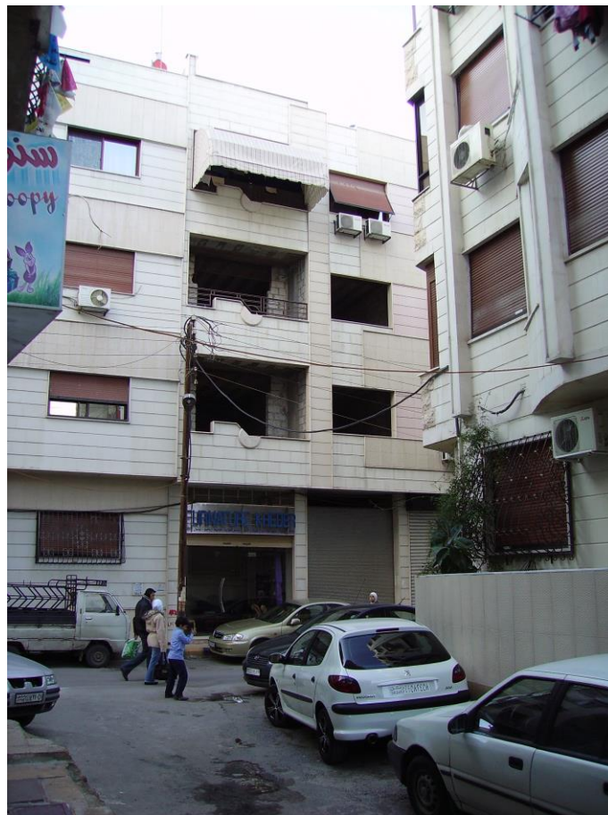
Caging windows at the first floor level for security reason on the right side by the A.C. and across the street next to the opened store (2010, by the author)
