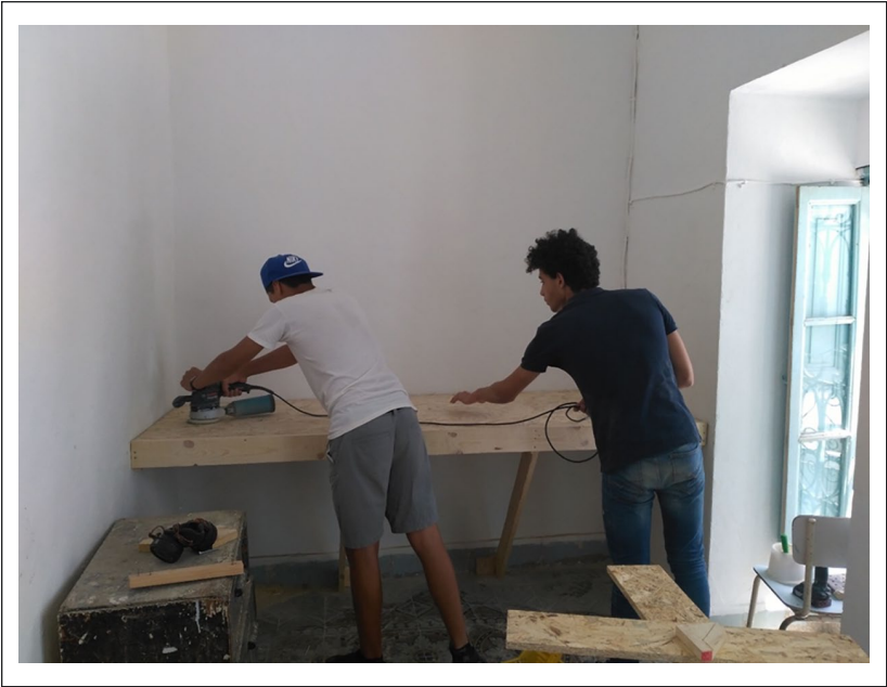
Figure 3. Building a work bench for Darna—2018.
